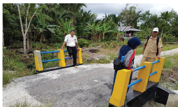
A newly constructed bridge for Tanjung Padang funded by a No Burn Village Reward.
